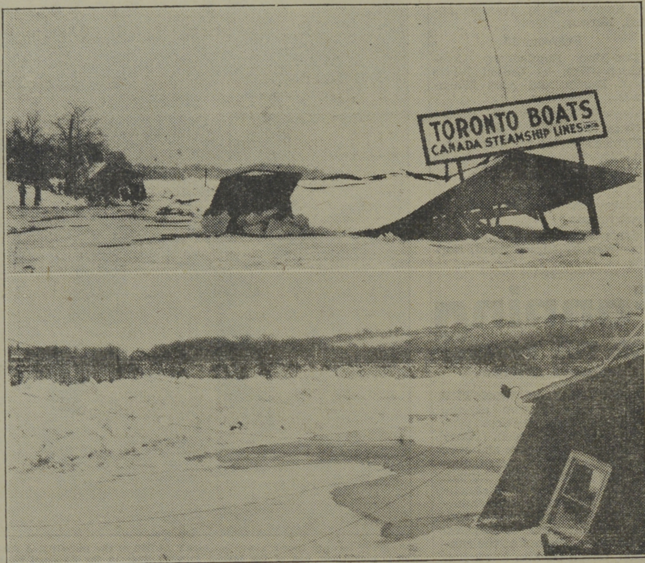
The havoc caused by the ice jam at Niagara Falls is shown in the above pictures, taken recently. At the top, the Canada Steamship Lines freight sheds have collapsed under the strain of thousands of tons of ice; while at the bottom, the former ticket office of the steamship company is tilting perilously while all around is ice and deep water.
