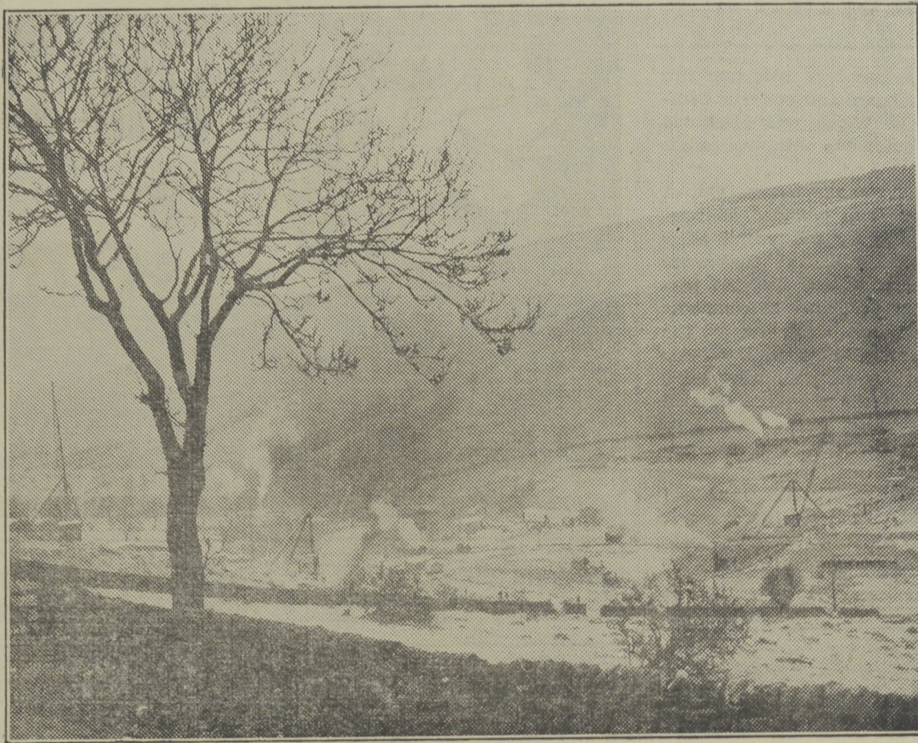
Work has begun in the construction of the new reservoir in the Derwent Valley, near Sheffield, England, and shows several steam shovels busy excavating near Ashopton. The new reservoir will eventually submerge
