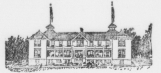
MUSKOKA FREE HOSPITAL FOR CONSUMPTIVES. MAIN BUILDING FOR PATIENTS.
