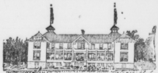
MUSKOKA FREE HOSPITAL FOR CONSUMPTIVES. MAIN BUILDING FOR PATIENTS.
