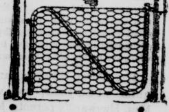
and covered with poultry netting. The hinges used were made of heavy wire bent in the way shown at Fig. A. The hook part fitted into a large screw eye fastened into the gate post. The gates are durable, cheap and easy to make and the idea might be utilized with profit by people who want to make attractive gates that will last.
