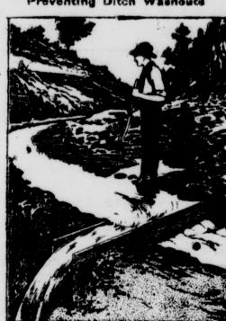
Spillways placed in irrigation and herdest experiences I ever had vent washouts during periods of high water. The spillways may be made of wood and should be placed as shown in the sketch, about one-fourth of a mile apart. The bottom of the trough should be grooved into the sides to make a substantial construction. Popular Mechanics.
