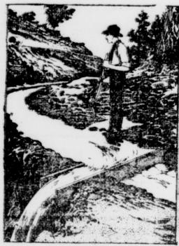
Spillways placed in irrigation and mining ditches on hilly ground prevent washouts during periods of high water. The spillways may be made of wood and should be placed as shown in the sketch, about one-fourth of a mile apart. The bottom of the trough should be grooved into the sides to make a substantial construction. Popular Mechanics.
