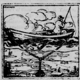
is fishing to swing around and continusually causing the line to become entangled with the anchor rope. This difficulty can be obviated by equipping the anchor rope with a bridle. The anchor being thrown out from the how of the boat and bridle rope is attached to the stern and adjusted to the other line as is suitable to the
