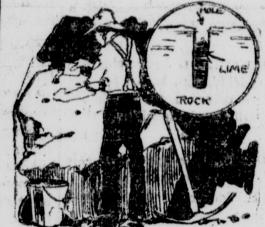
gry wooden plug into the hole and mas water on h. The expansion of the wood will cause the rock to split
