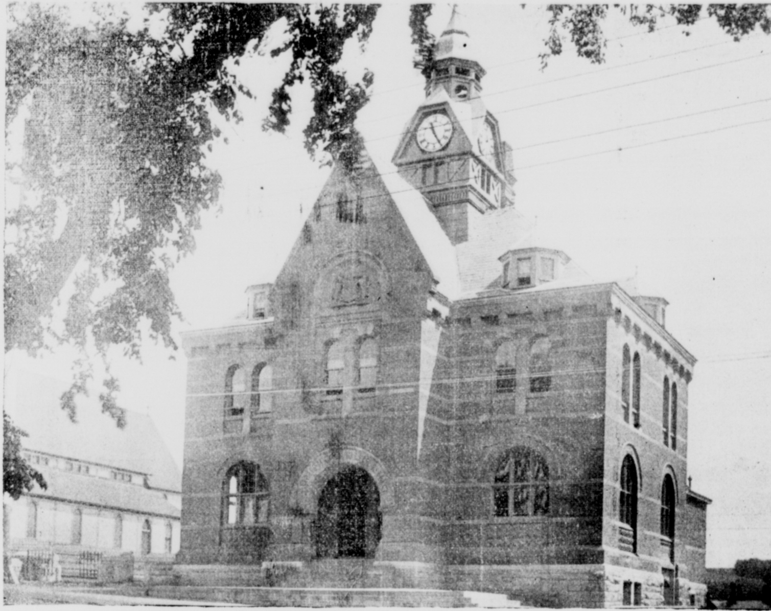
POST OFFICE AND CUSTOM HOUSE.
