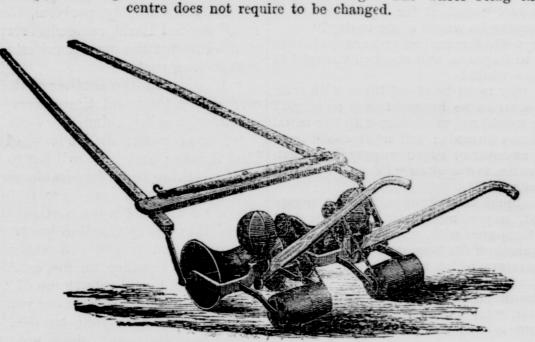
Bell's One Horse Double Drill Seed Sower. For sowing root seeds of all kinds. Sure sower and no loss of seed when turning sowing only one drill. Rolls and drill before sowing, puts the seed into the ground, covers and rolls after sowing, all at one operation. The quantity of seed to be sown is easily regulated by a slip band on the seed canister. The Seed Drill is very low in price,
