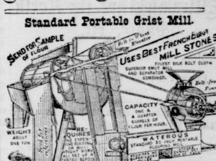
Specially adapted to the wants of the Maritime Provinces. WM. CURREY, writes from Windsor, N. S., Dec. 79. "The 20 inch Standard Flour Mill works satis factorily. The smut mill cleans well. The 12 meh Standard chops 12 bush. per hour. The far-
