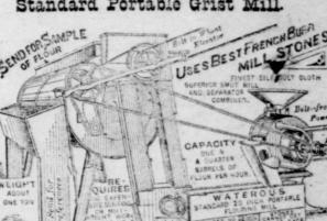
Specially adapted to the wants of the Maritime Provinces. WM. CURREY, writes from Windsor, N. S., Dec., '9. "The 20 inch Standard Flour Mill works satis factorily. The smut mill cleans well. The 12 inch Standard chops 12 bush. per hour The far-
