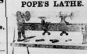
For Turning, Boring, Drilling, Grinding, Polishing, Scroll and Circular Sawing, And all purposes for which a Lathe is intended.
