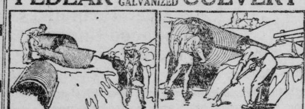
These pictures show how easily and cuickly you can lay Pedlar Culvert. Comes nested, half-section within half-section---saving freight and cartage. Triple-thick Flat flange locking ribs on each side are clamped together by a simple tool---no bolts nor rivets needed. Joints are broken---only culvert you can do that with. Ends interlap. Will stand tremendous strains. Won't leak, nor buckle, nor crack from frost. Cheaper than wooden culverts
