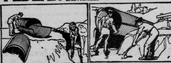
These pictures show how easily and quickly you can lay Pedlar Culvert. Comes nested, half-section within half-section---saving freight and cartage. Triple-thick Flat flange locking ribs on each side are clamped together by a simple tool---no bolts nor rivets needed. Joints are broken---only culvert you can do that with. Ends interlap. Will stand tremendous strains. Won't leak, nor buckle, nor crack from frost. Cheaper than wooden culverts
