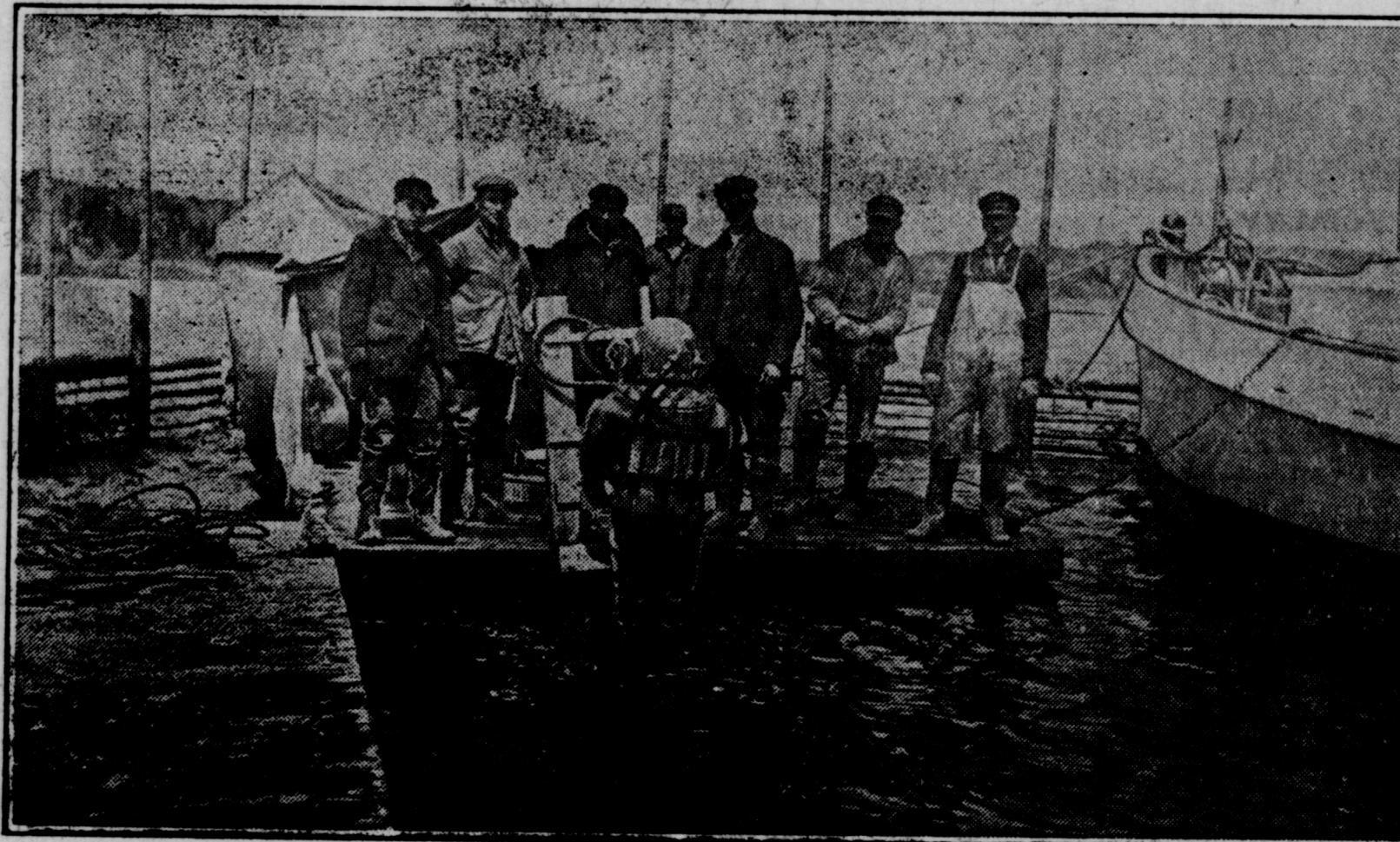
A DIVER AT WORK—CLEANING THE BOTTOM OF A WEIR—A NECESSARY AND EXPENSIVE WORK.
