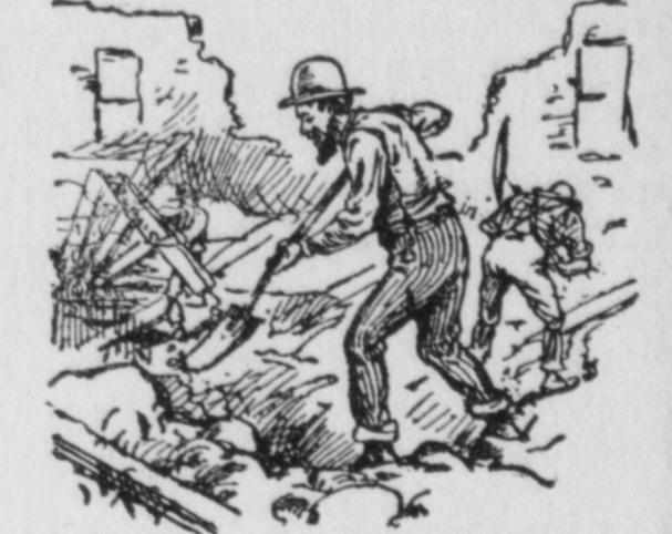
"I was helping dig out the cellar."
