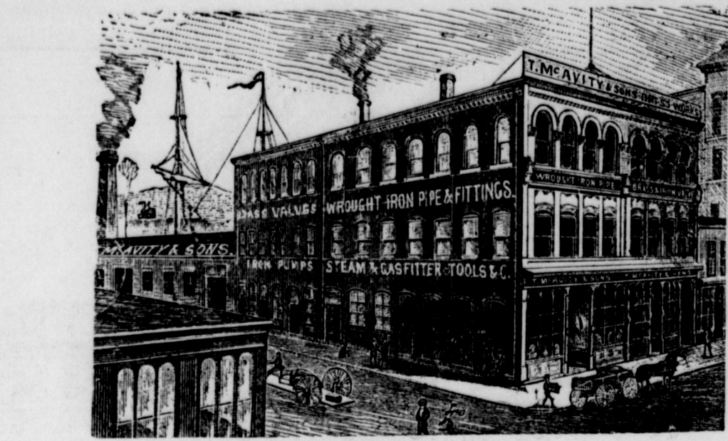
THE FACTORY ON WATER STREET.
