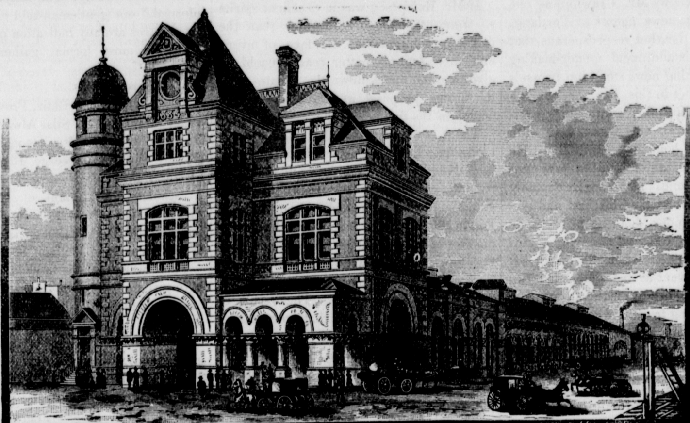
SAINT JOHN PASSENGER STATION.
