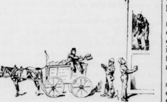
PASSING BRICKS FROM CART TO SECOND STORY OF HOUSE.
