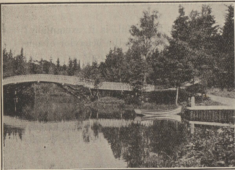
BRIDGE OVER ARTIFICIAL LAKE
