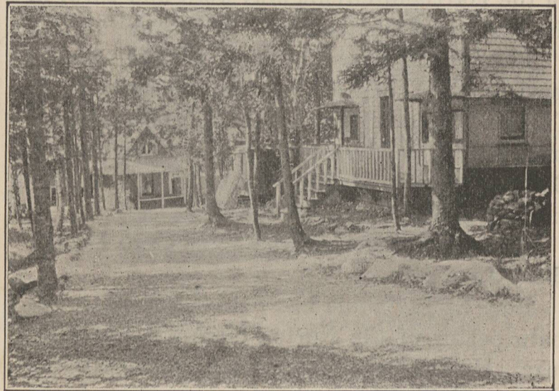
A section of Kinghorn Avenue near the bend.
