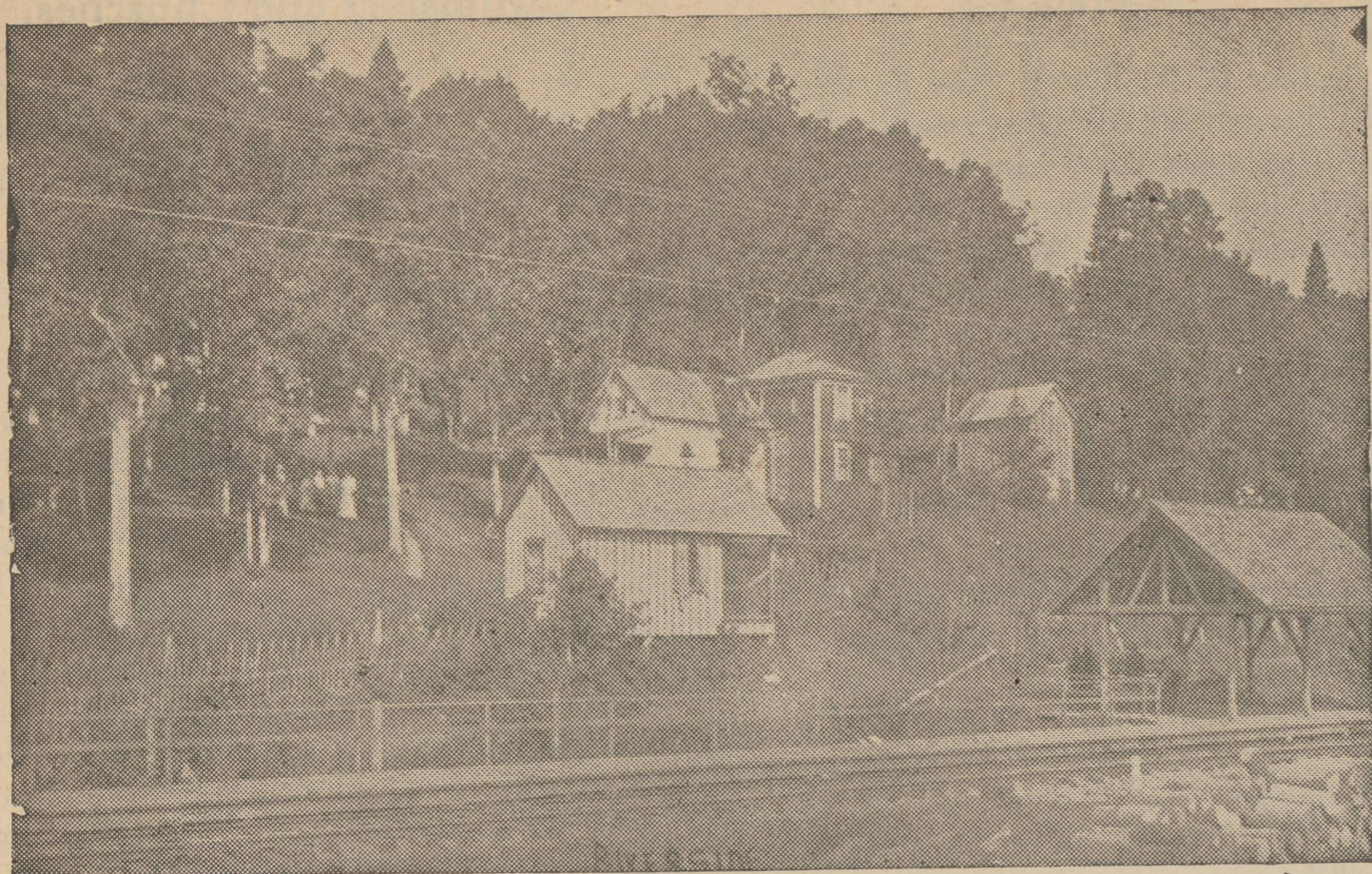
RIVERSIDE CAMP GROUND, ROBINSON, MAINE
