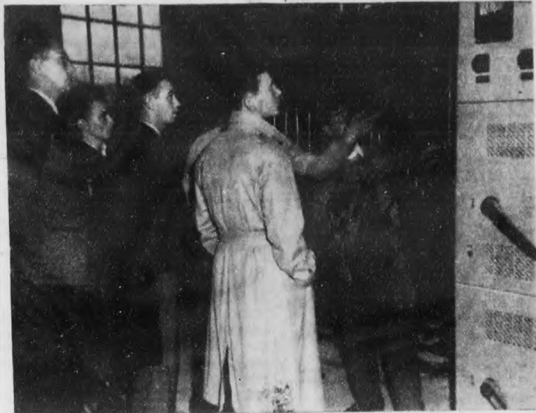
Electricals inspecting transformer banks and switchboard at the Fraser Paper Mill in Newcastle, N. B., during the engineer's first field trip last fall. Left to right: Jack White, Maurice Cyr, Ross Wetmore, Don Prendergast, and Doug Stewart.
