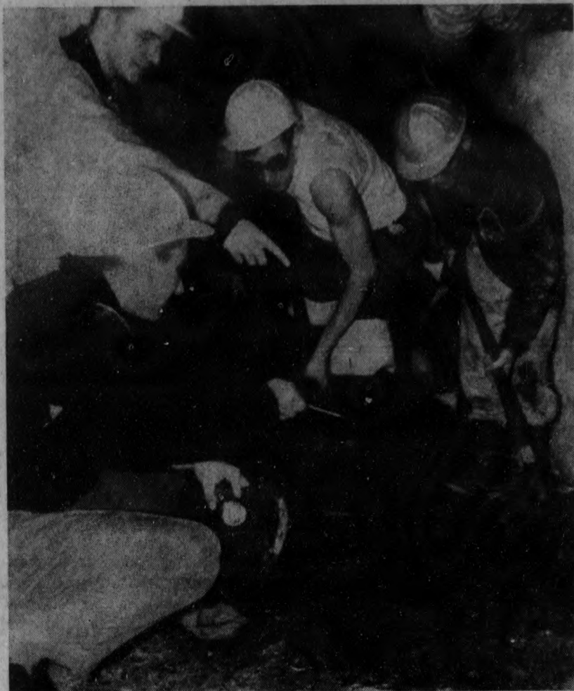
MEN FROM LBR BEGIN EXCAVATIONS ON NEW TUNNEL TO LADY'S RESIDENCE
