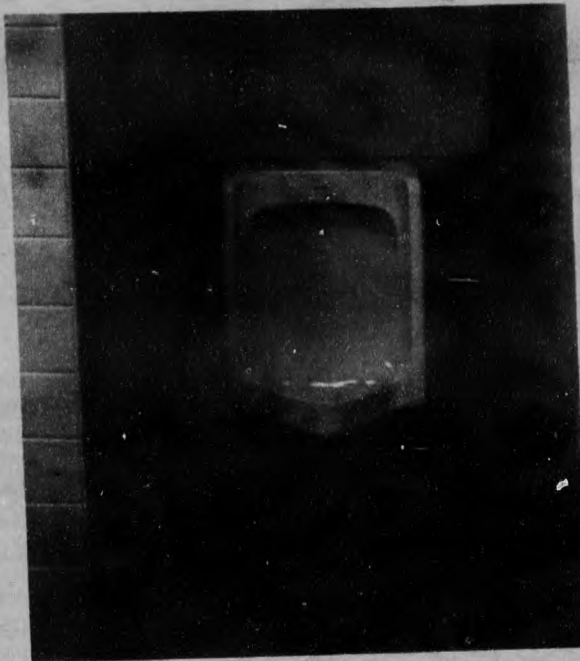
(b) above the urinal - speed and efficiency
