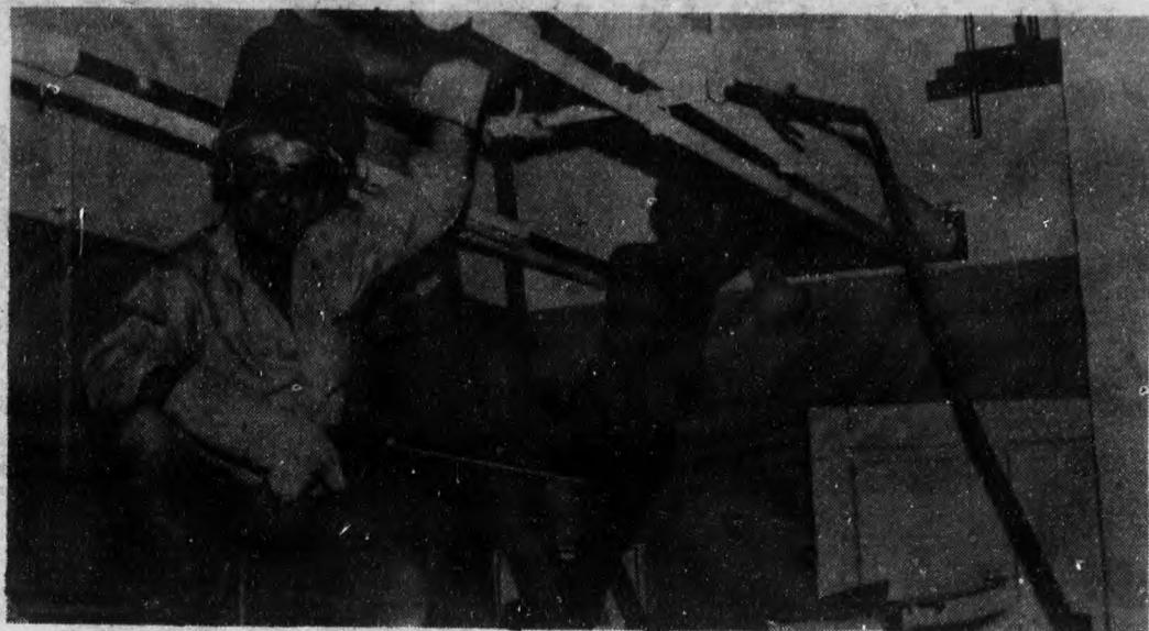
Here workers show how it's done as they rebuild Lady Beaverbrook Residence.
