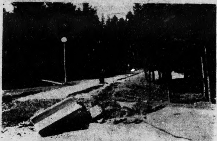
Work on a roadway behind the SUB began last week. The road will carry traffic from the SUB's traffic circle to the Law Building.
