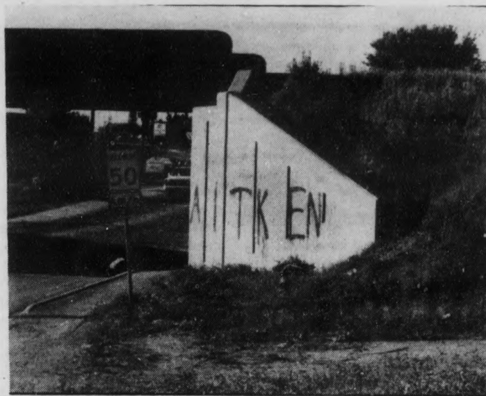
Underpass hit by Aitken painters
