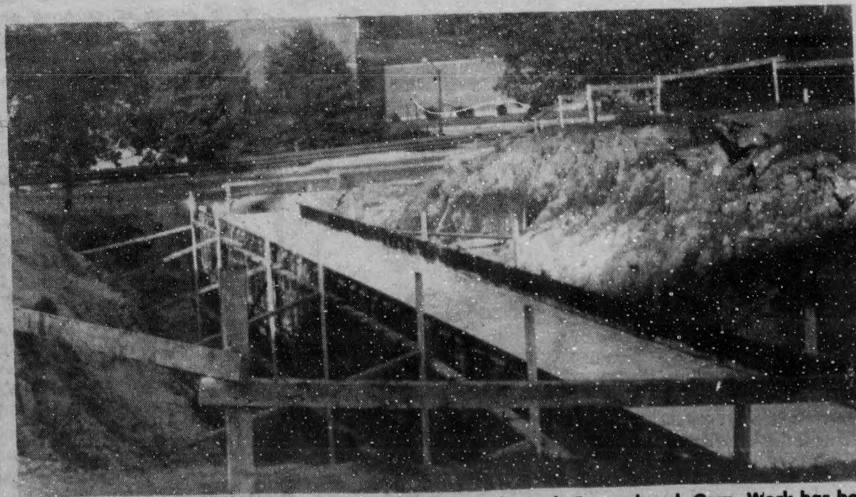
To cure the problem of leaky steam pipes leading to the Lady Beaverbrook Gym, Work has been going on over the last few weeks to install a new tunnel. The work should be finished by the end of October, but while it is in progress it will be necessary to close the road for a while in the next couple of weeks.
