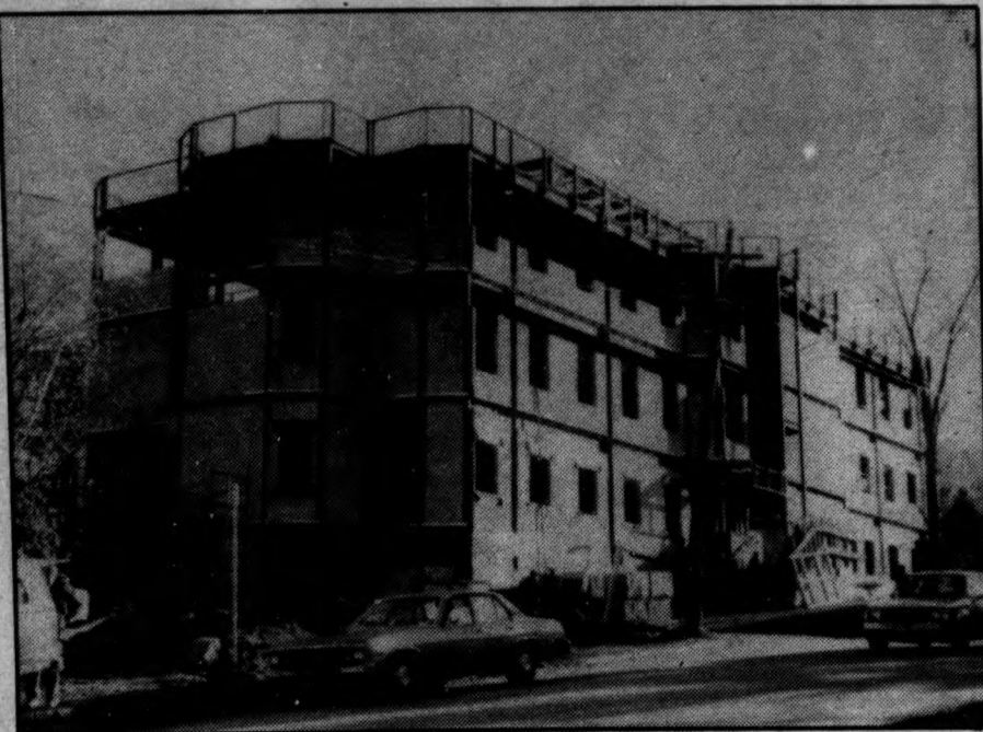
Head Hall presently under construction
