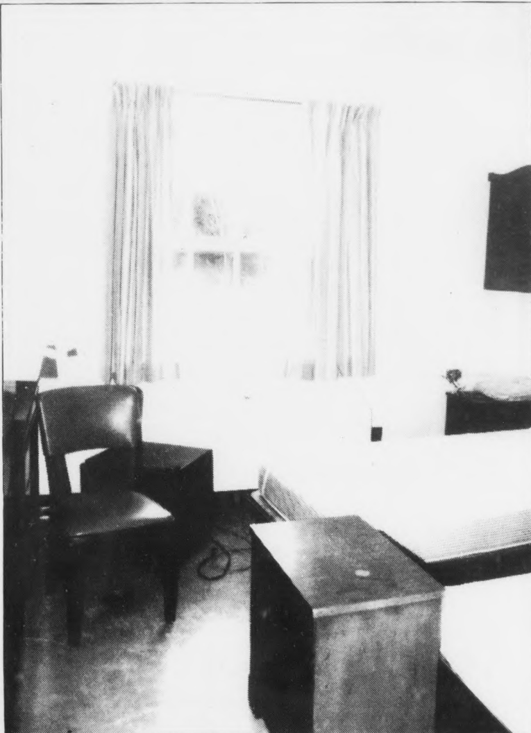
Shown is one of the rooms damaged in the fire at Lady Dunn Hall on November 15, 1992. Restoring the residence could cost the university up to $200 000. Kevin G. Porter photo.
