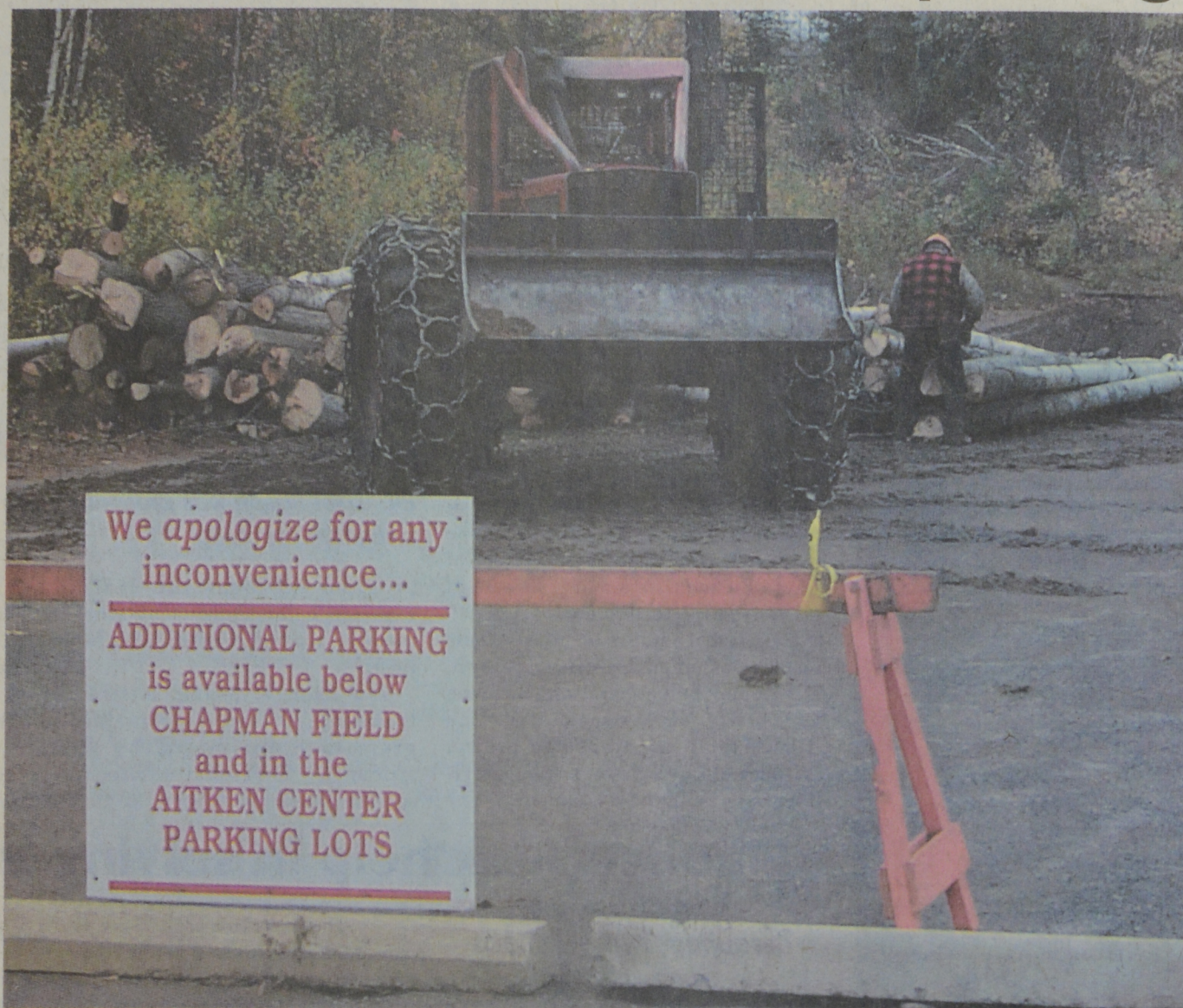
Construction on the National Research Centre at UNB began on Wednesday.
