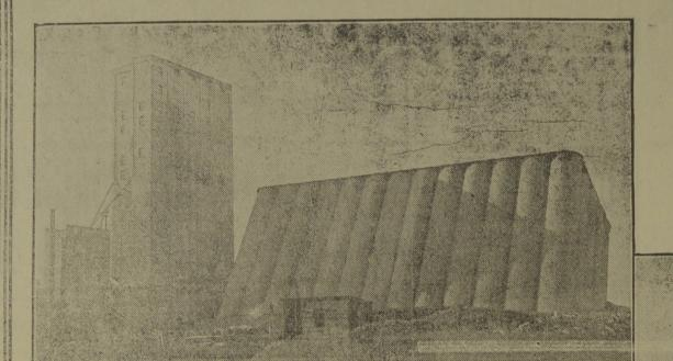
Views of both sides of the million bushel C.P.R. Concrete Grain Elevator at Transcona, Man., which recently settled on its foundations and now stands intact at an angle of 30 degrees.
