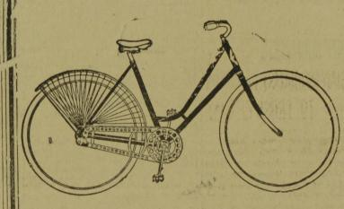
Coaster Brake Mud Guards **Studded Double Tube Tires** Extension Handle Bars
