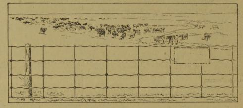
A strong and serviceable fence, a popular style and easy to erect. All made of No. 9 Galvanized wire and tightly interlocked. Remember the price-58c. per rod, freight prepaid to your nearest railway station or boat wharf.
