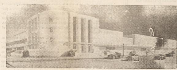
The latest in radio engineering and studio construction progress is embodied in these new National Broadcasting Company studios being constructed in Hollywood. Departing radically from the conventional radio center design, the new studios are patterned after the motion picture plan. There are four large individual studios under separate roofs, each seating several hundred persons, and four other studios without audience accommod
