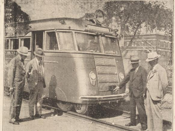
THE first tests to be made in Canada of a new type of automotive vehicle which links highway and railway will be commenced within the next two weeks on branch lines in the three regions of the Canadian National System. The first of these "Auto-Railers" which will be tried out on branch lines in Ontario and Quebec, is now ready for service. It was inspected recently by S. J. Hungerford, Chairman and President of the Canadian National, and a number of headquarters officials.
