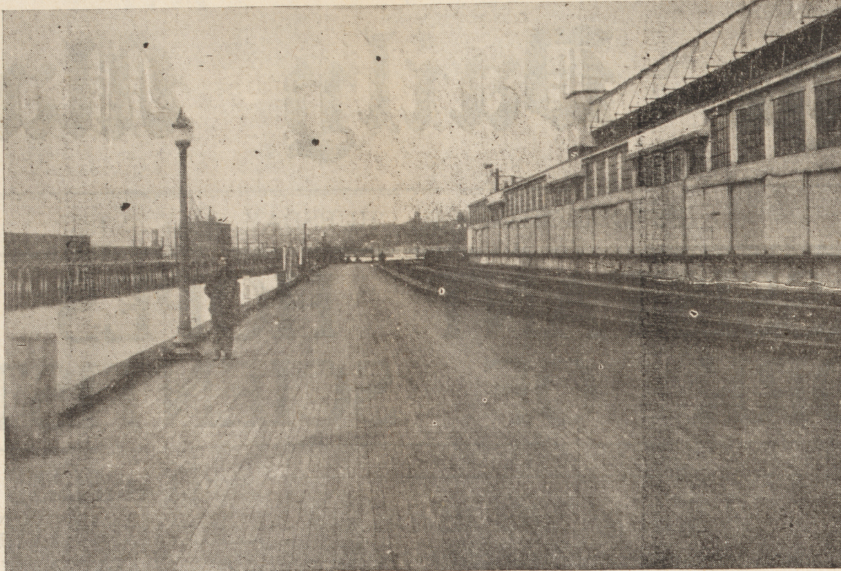
CREOSOTED HARDWOOD DECKING USED IN DRIVEWAY TO NO. 7 SHED, SAINT JOHN HARBOR, OVER 150,000,000 FEET OF HARDWOODS HAVE BEEN CREOSOTED IN TWO CREOSOTING PLANTS ESTABLISHED IN NEW BRUNSWICK.
