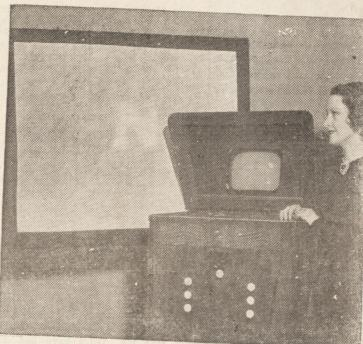
The White area in this picture is the screen on which RCA television was shown for the first time during a practical demonstration from the NBC television studio in Radio City. Betty Goodwin, NBC television announcer, stands alongside a regulation television receiver, which shows an image sevenand-a-half by ten inches compared to the screen picture of approximately three-by-four feet.
