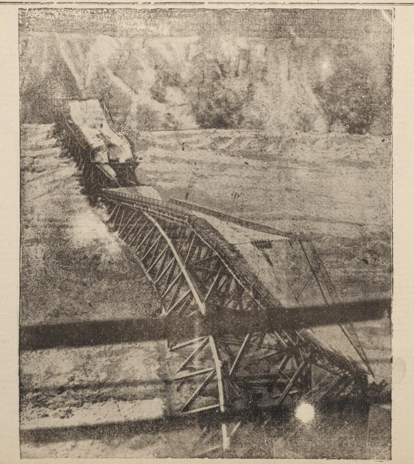
This picture, taken a moment after the Falls View bridge fell into the Niagara River gorge recently, shows the power of Nature when it is exerted. The 39-year-old structure was torn from its abutments and the steel twisted and torn apart. It is still lying on the ice jam.
