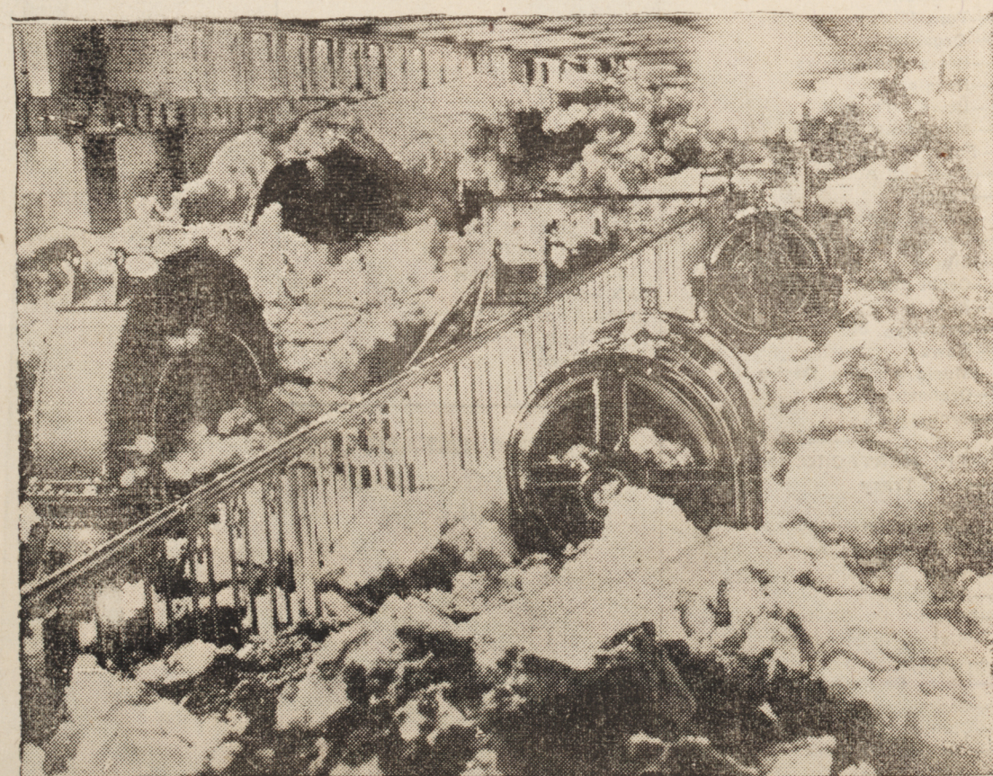
Niagara's losses from ice, the worst in two generations, were not all confined to the collapse of the Fallsview ("Honeymoon") bridge. The $16,000,000 plant of the Hydro-Electric Power Commission of Ontario was overwhelmed by cakes of frozen spray and water as shown herewith and one battery of the huge generators will be out of business for several weeks as a result.
