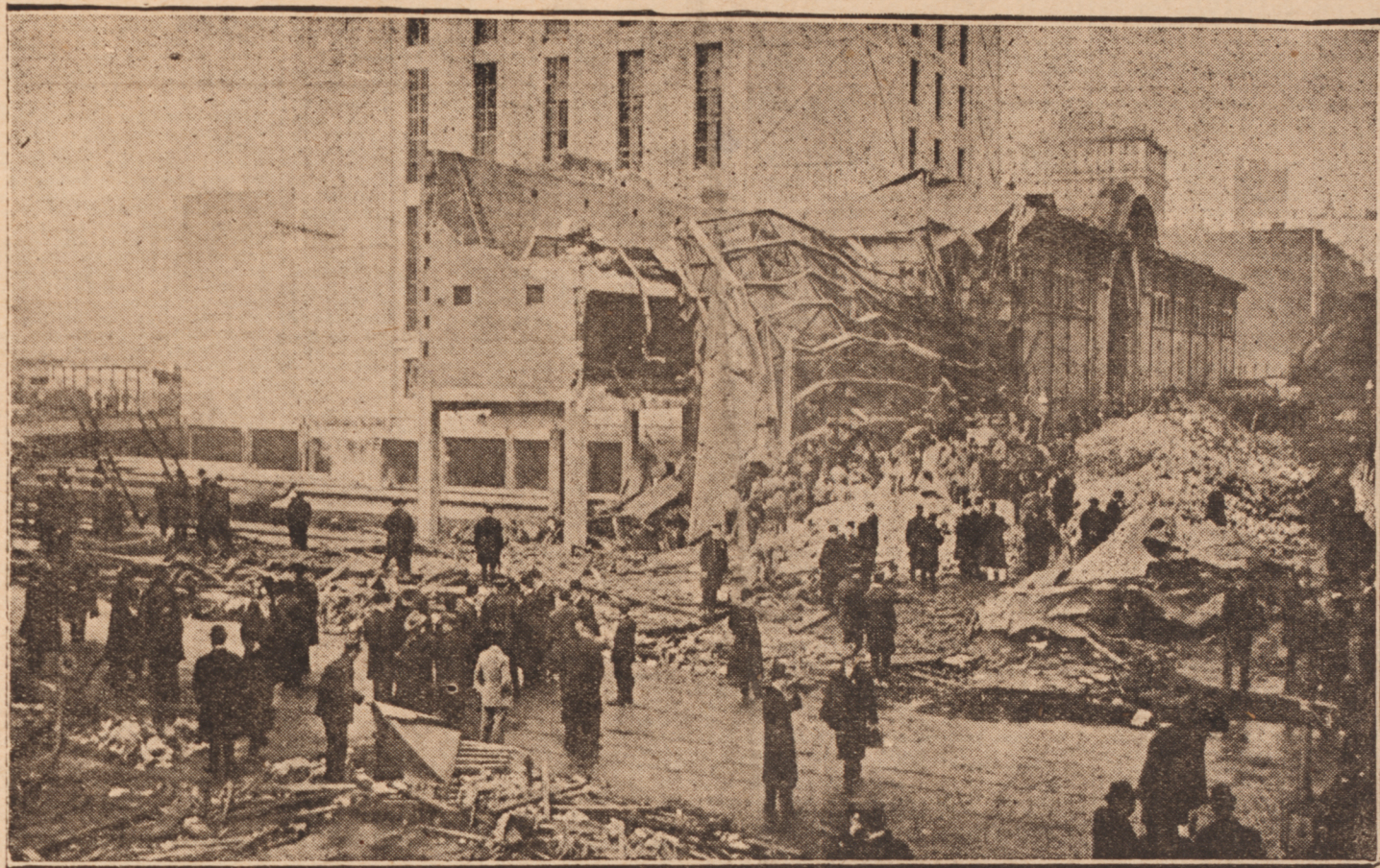
New York, Dec. 27.—The above illustration gives some idea of the extent of the explosion which caused the death of ten persons, the injury of 106 and damage to property to the extent of $270,000 in the powerhouse of the New York Central Railroad, at Lexington Avenue and Fiftieth Street, New York. Pedestrians were hurled from their feet to the sidewalk or sent bruised against the houses. Many rushed into places of shelter holding their hands to wounds on their heads and faces. A policeman was leading a twelve-year-old girl across the street, when one of her feet was nearly cut off by a flying fragment of glass. At every hand were strange manifestations of the irregular action of the force which the explosion had released.
