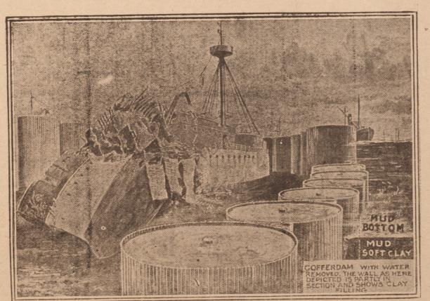
WRECK OF THE MAINE AS IT WILL BE WITHIN WALL OF COFFERDAMS AFTER THE PUMPING OUT OF THE WATER FROM THE SPACE THUS ENCLOSED HAS TAKEN PLACE.
