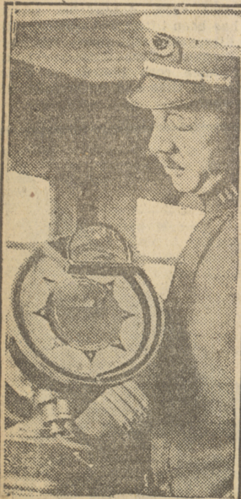
"Metal Mike" is the name given the automatic steering gear of a steamship Marengo. This mechanical device keeps the ship on its course. The Marengo sailed to the West Indies and back with Metal Mike doing the
