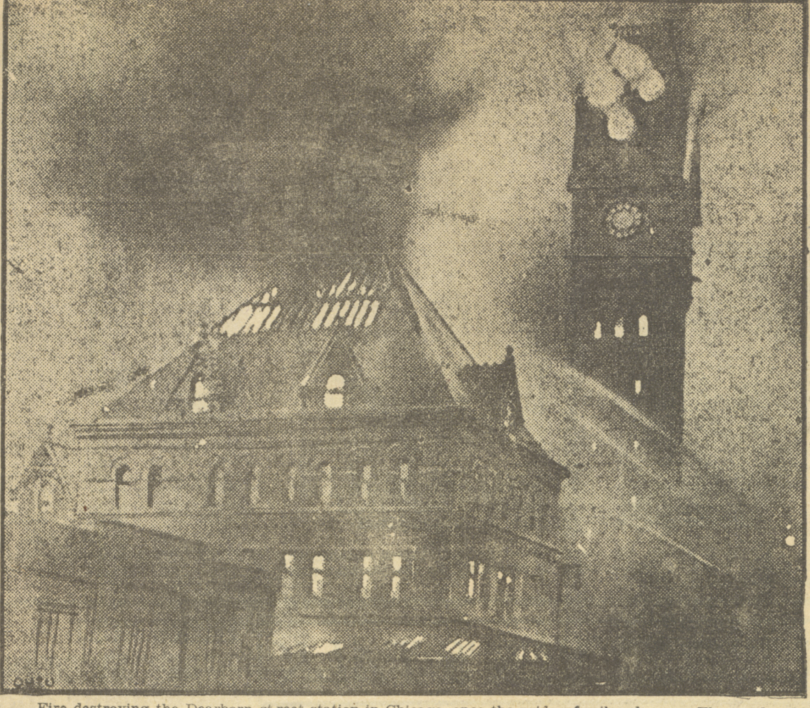
Fire destroyed the Dearborn street station in Chicago, once the pride of railroad men. The wood and brick structure crumbled easily beneath flames which started, it is believed, from crossed wires. It cost $300,000 to build the depot; it will cost $1,000,000 to rebuild it, say architects.
