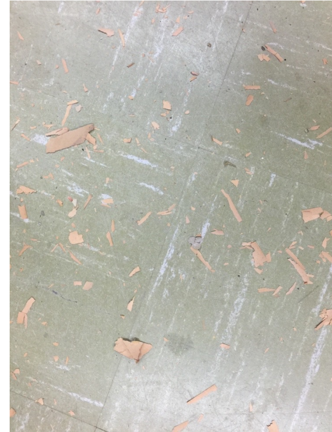
the floor after imaging
